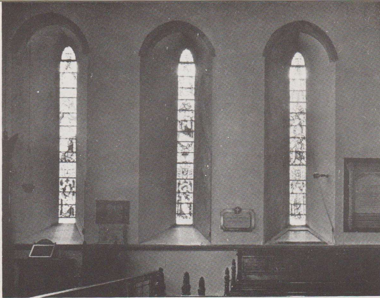
Three of the five 12th century lancet windows, showing some of the original stonework and 12th century decoration. These windows were discovered and restored in 1894.
