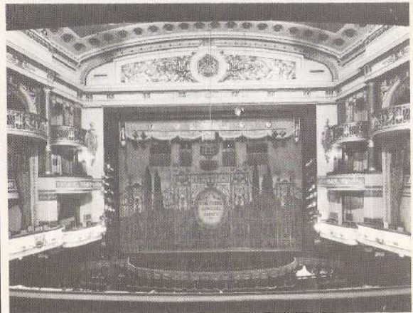
The interior of the theatre
